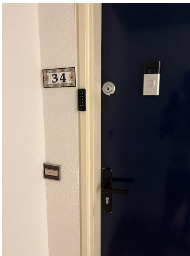
Entrance door, keypad on the left
